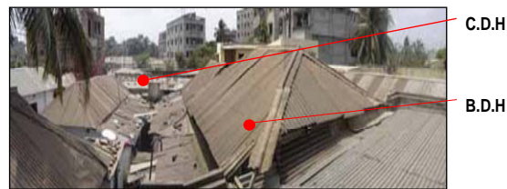
Figure 3. Physical position of the Bangladesh Traditional House (B.D.H) and the Contemporary Design House (C.D.H).
