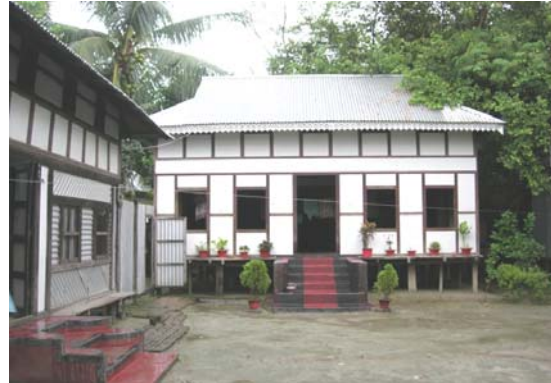
Figure 2. Typical Bangladesh Traditional House.
