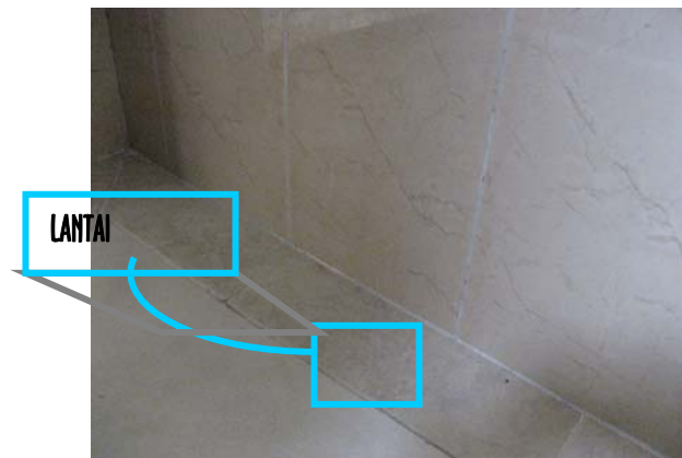
Gambar 4.14. Lantai Kamar Mandi
