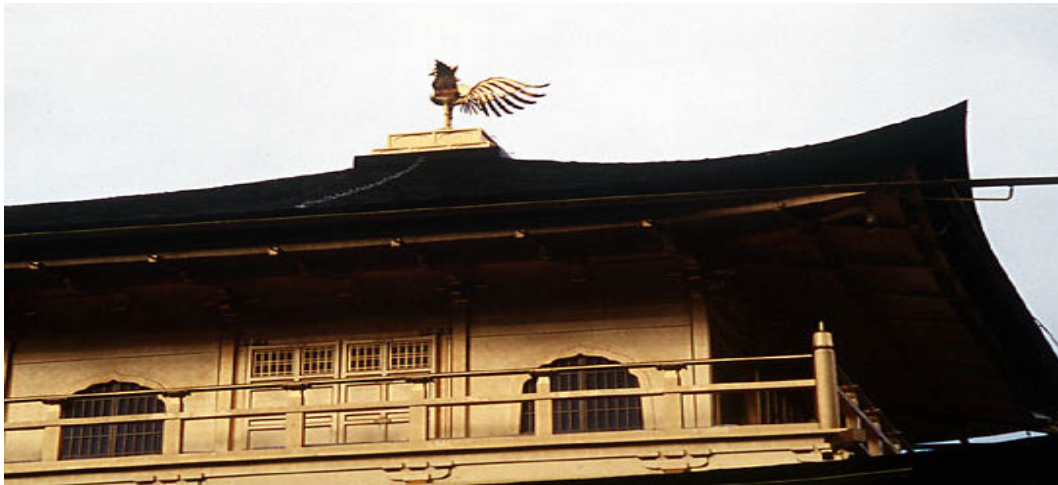
Detail of the roof and upper storey, designed in the Zen style with cusped windows.
