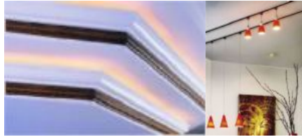
Gambar 2.28. Linear Lighting System
