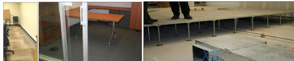
Gambar. 32 Underfloor Air Distribution System.
