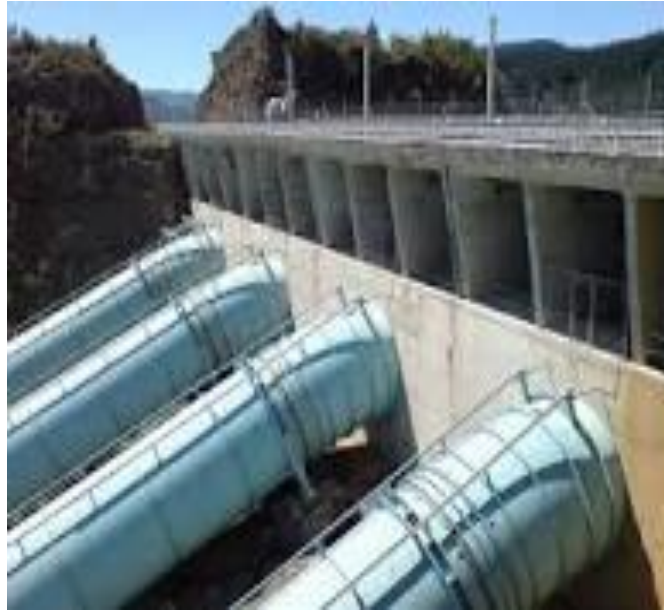
Gambar 2.6. Pipa Pesat ( Penstock )
